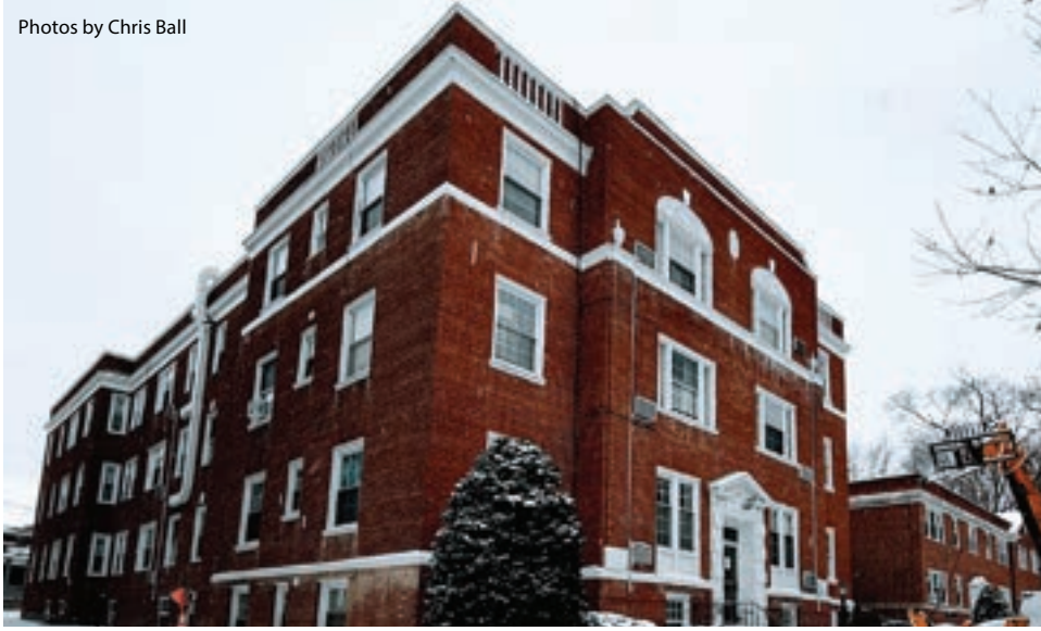
This apartment building at 13654 Fairhill Road was evacuated in early January first for no heat and then for no water.
