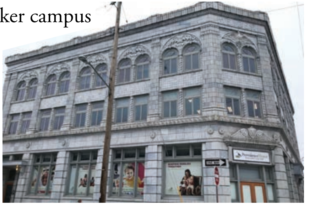
Providence House renovated the vacant Weizer building on Buckeye Road for its new East Side campus, called Hope's House. Photo by Chris Ball
