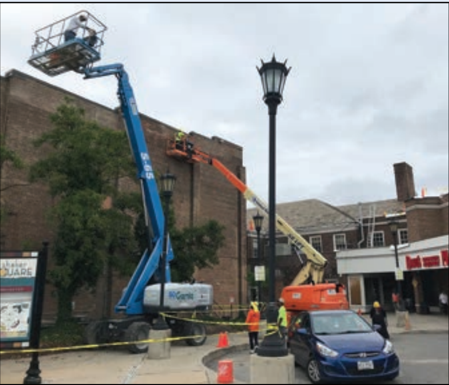
Workers on cherry pickers raise up high in the sky for tuck pointing of the brick wall behind Atlas Cinemas on Sept. 8, part of the restoration work taking place at Shaker Square.
