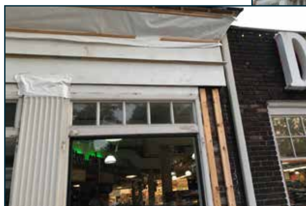
Work continues on the façade of Dave's Market on Shaker Square.
